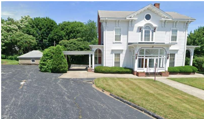
Image 1: Existing Structure at 36 Butler Street (Google Streetview, June 2023)
